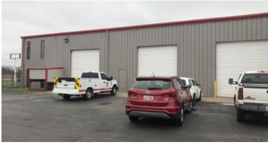
Figure 115: SC-ESD 2 Fleet Maintenance Facility
